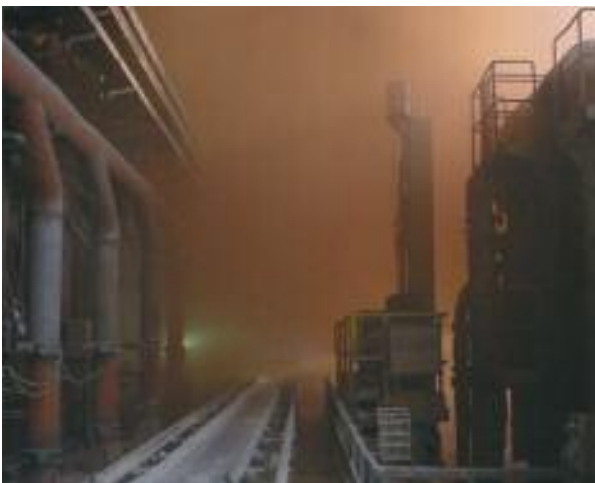
Series 4040R in steel works environment - Travel 34.5 ft (10.5 m), Speed 197 ft/min (60 m/min), Fill weight 4.09 lbs/ft (6.084 kg/m)
