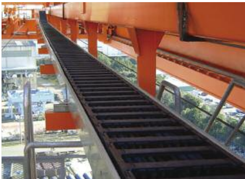
Long travel with igus® steel guide trough and harnessed igus® E-Chain® on a crane
