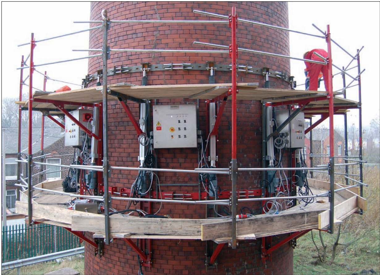
Adjustment of maintenance platform via SLZ 90 heavy duty cylinders.
