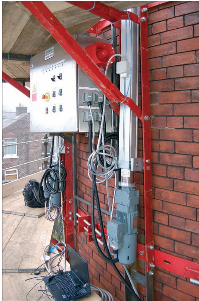
Adjustment of maintenance platform via SLZ 90 heavy duty cylinders.
