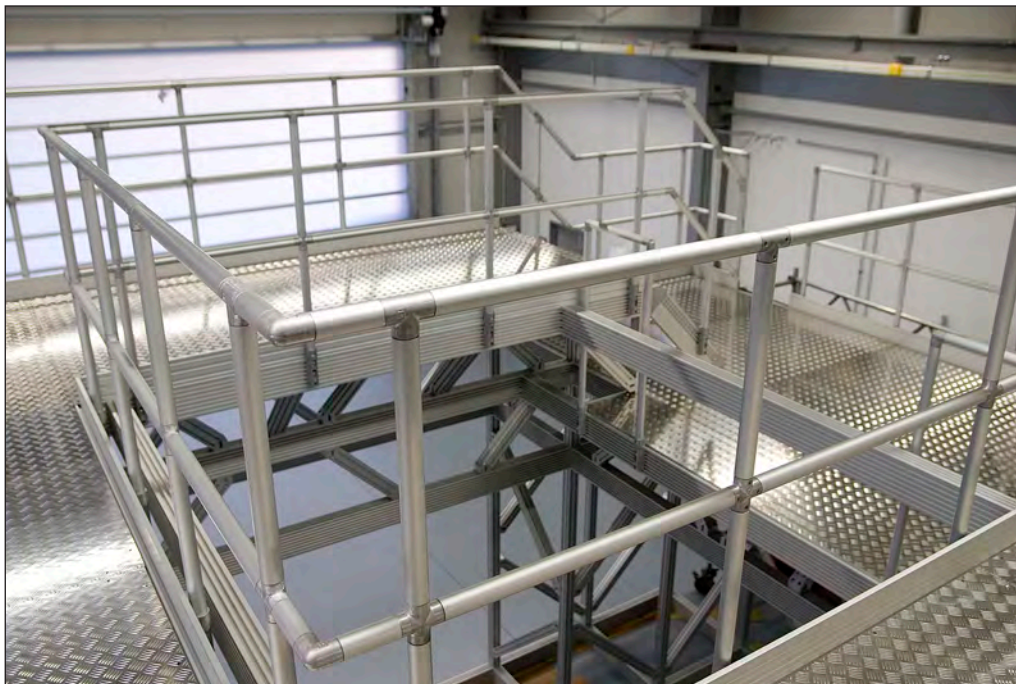
Working platform with ITAS railing
