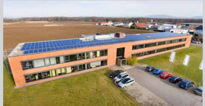
We take environmental protection very seriously: solar collectors on the roof of our building in Gottenheim generate more electricity than is required by the works.
